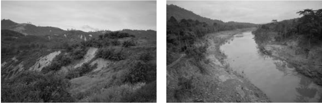
Figure 1: Landslide and slope failures at Hulu Sungai Galas (Left). Erosion and slope failures along Sungai Lebir Riverbank (Right).
