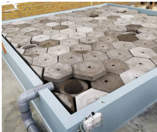
Figure 1: Field test for home-based StormPav green pavement system
