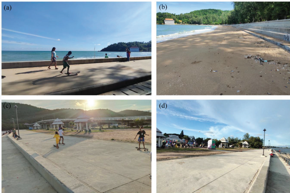
Figure 10: Stepped revetments in Thailand, designed by the authors: (a) The Laem Sadet beach, Chanthaburi province, Thailand, (b) The wide beach berm in front of the revetment at the Laem Sadet beach, Chanthaburi province, Thailand, (c) The Khaem Nu beach, Chanthaburi province, Thailand and (d) The stepped revetment at the Khaem Nu beach, Chanthaburi province, Thailand as a new tourist destination
