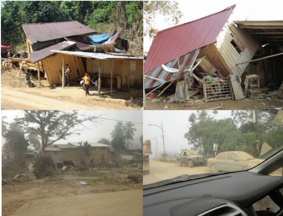
Figure 1: The aftermath of the Kelantan Big Yellow Flood of 2014 (self-collection)
