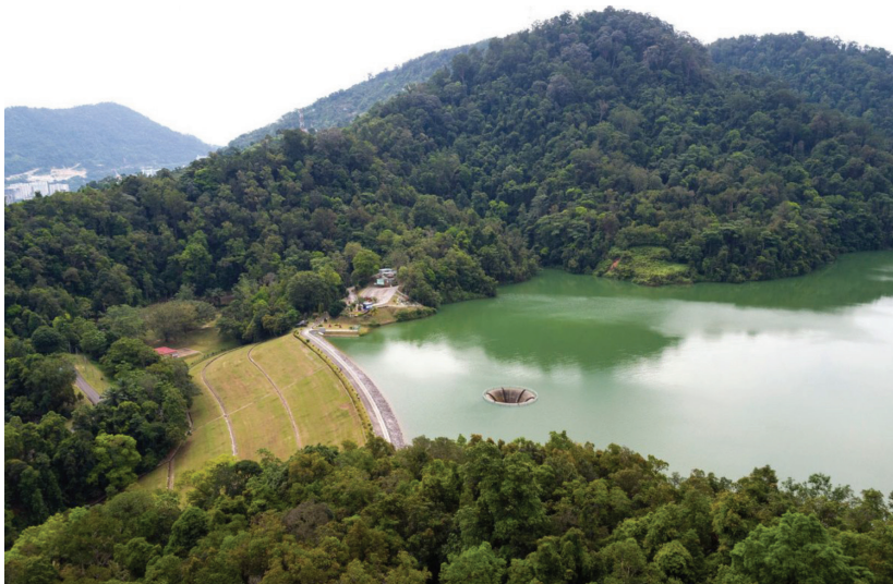
Figure 3: Air Itam Dam today
