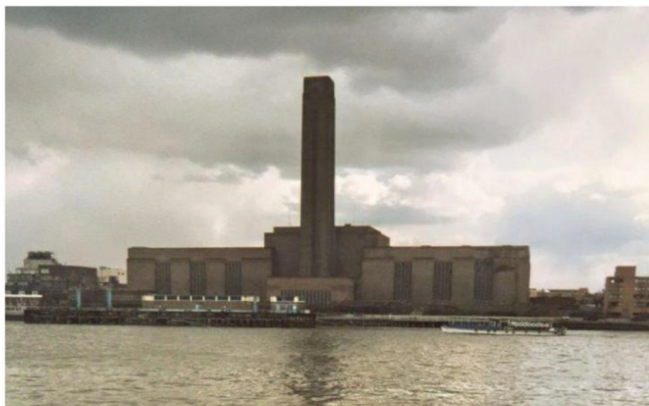
Figure 2: The Bankside Power Station Source: Wikipedia
