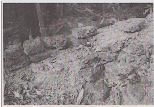
Figure 1: Candi structure made of laterite bricks is used as candi structure at Bukit Choras (Zakaria, 1989)
